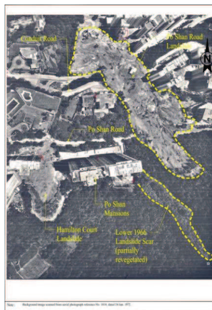
Figure 4: 1972 Po Shan Road and Hamilton Court Landslides
